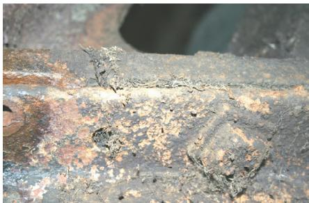
It was a shock to find in March 2007, on doing some regular maintenance, that the top tier of the frame had a couple of severe cracks close to a part of the frame that had already been plated. Ringing was suspended and quotations were sought to put the bells back in ringing order. It was even more of a shock to find that nearly £15,000 would be needed to get the bells and fittings back in good order.
